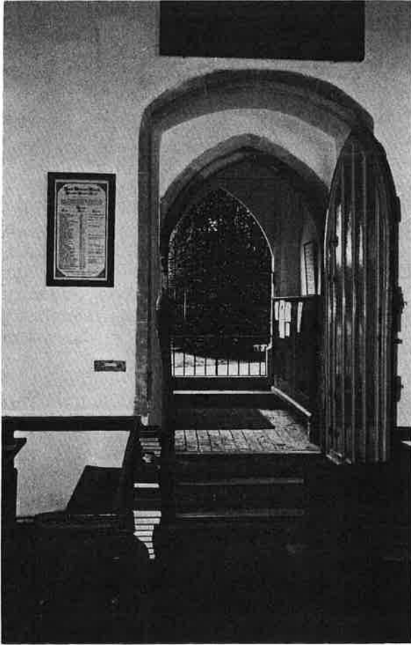
Looking up and out through the South door.
